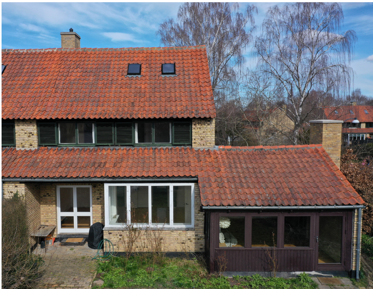
Facade mod haven Granholmen 26 (plads 3)
